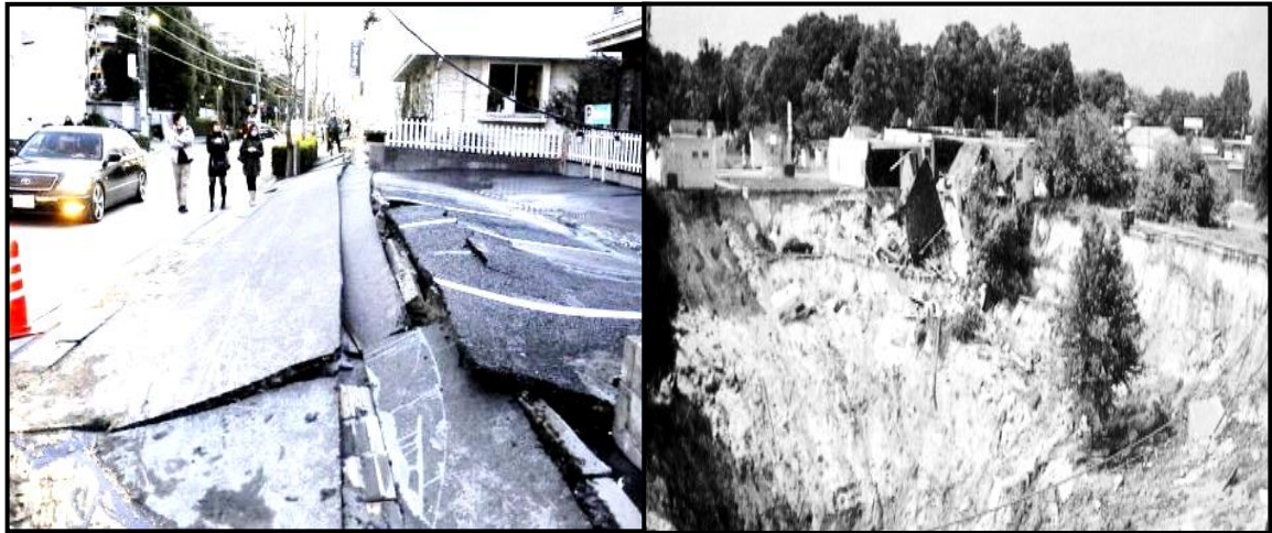
Earthquake cracking pavement and exposing underground rocks
