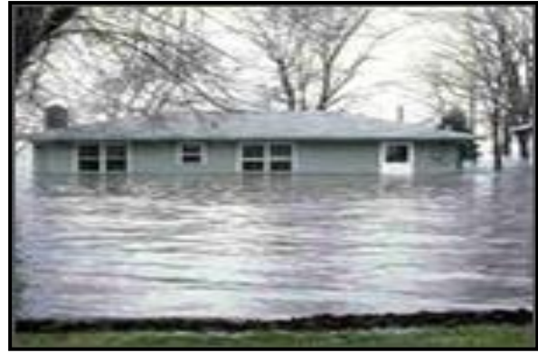
Building under water after a flood.
