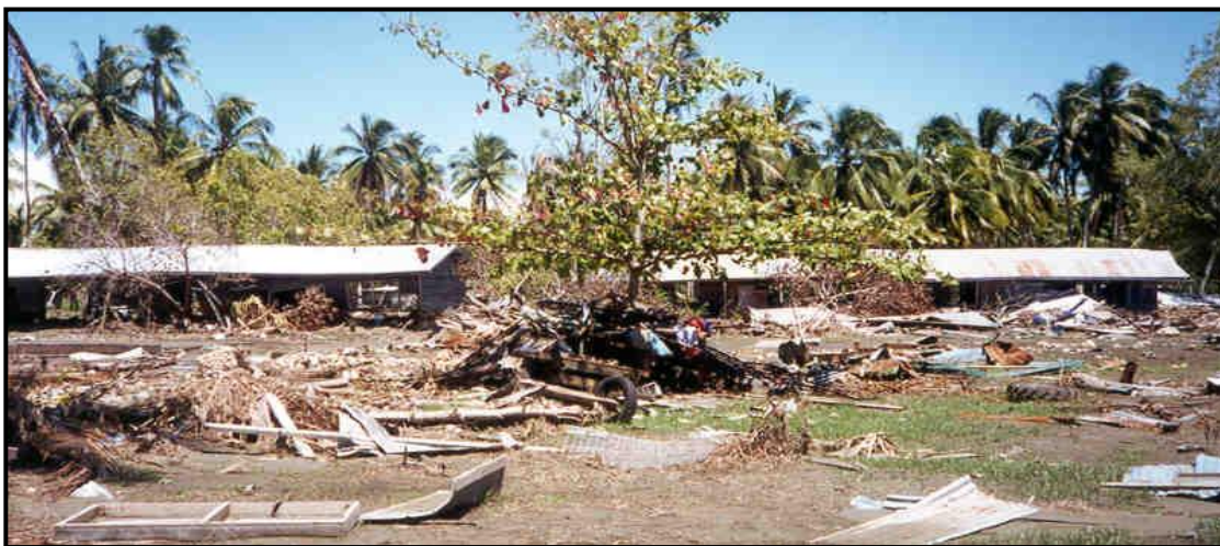
Damages caused by tsunami
