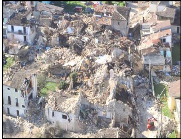
Great destruction caused by an earthquake
